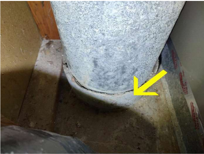
metal transitions to transite @ floor slab
